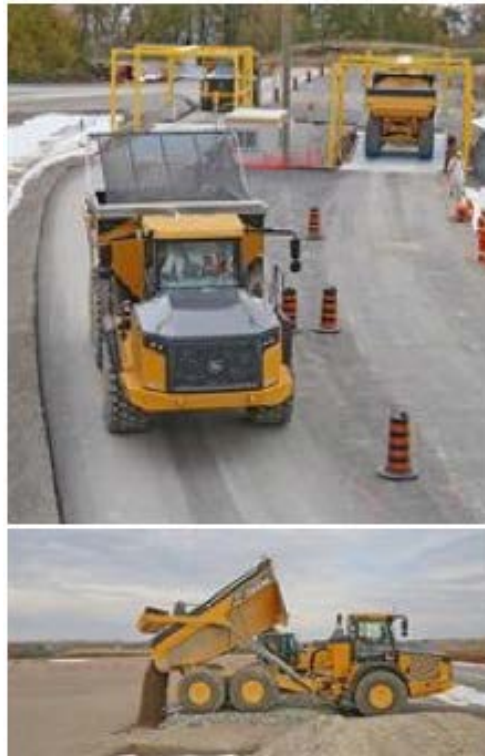
Figure 6: Transfer of Waste to the Newly Constructed LTWMF on Dedicated Haul Road
