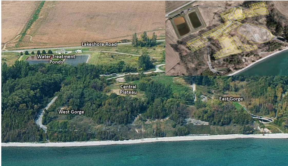
Figure 3: Existing Port Granby Waste Management Facility on the Shore of Lake Ontario (insert - Layout of Burial Trenches)
